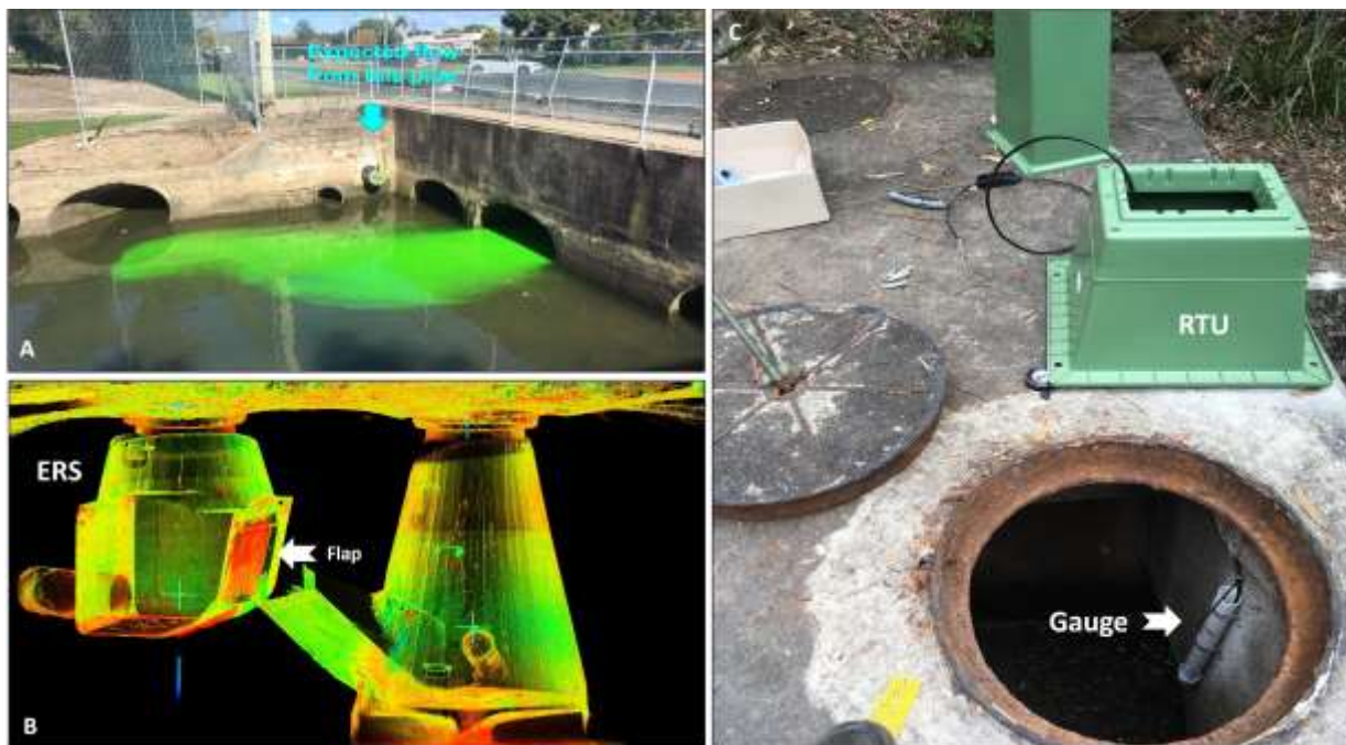
Figure 7-6: (A) environmentally sustainable dye used to locate ERSs; (B) 3D image of an ERS; and (C) configuration of a sewer gauge and RTU
