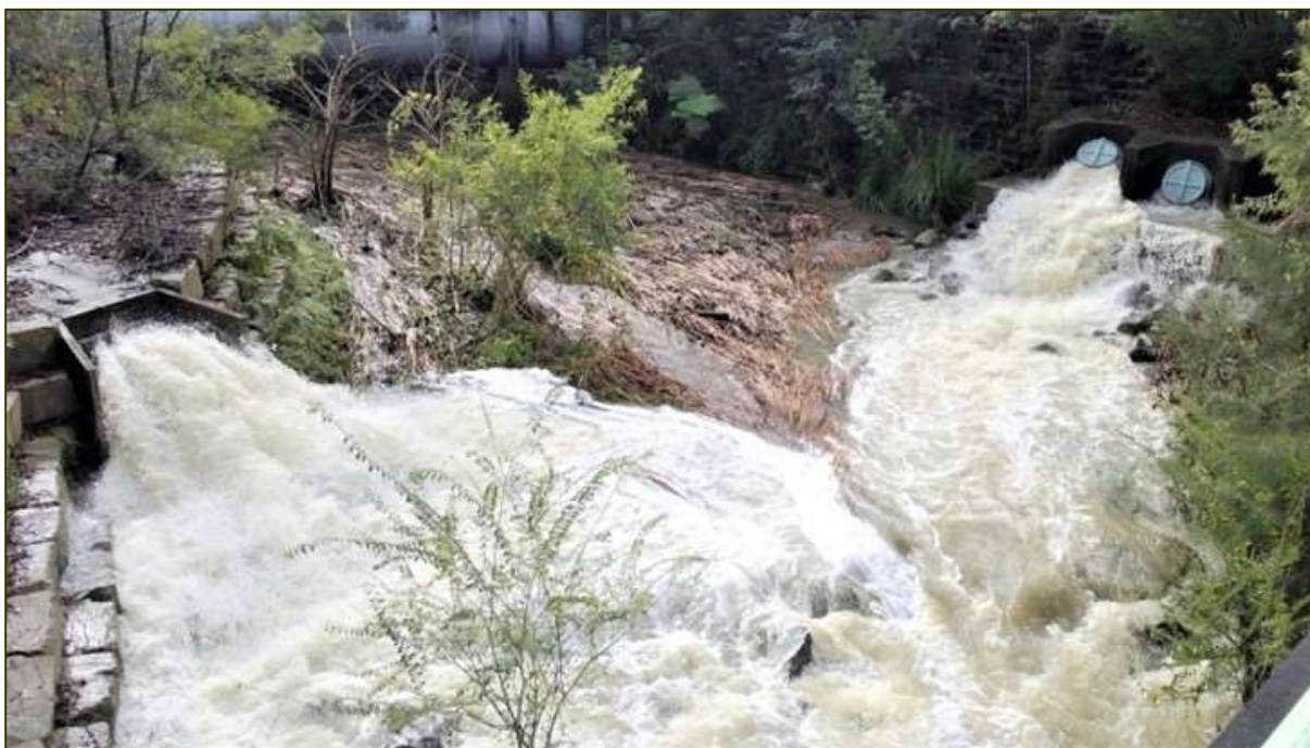
Figure 4-5: Three adjacent ERSs spilling influent into Vineyard Creek and stormwater flows
