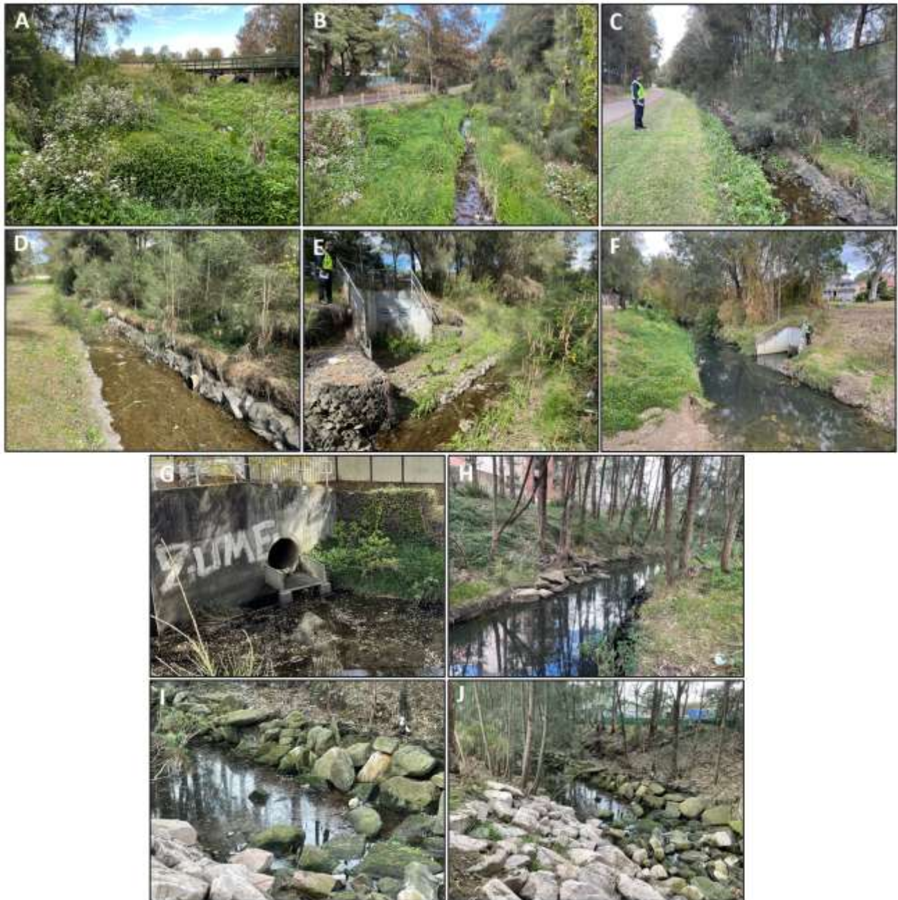
Figure 4-21: Images of Girraween Creek on a day after 5 mm of rainfall the night before the visit Girraween Creek: (A) upstream site; (B) 500 m below upstream; (C) 750 m from upstream site; (D) about 1 km from upstream site (E) 600 mm duckbill ERS mid-way toward downstream site; (F) 600 mm duckbill ERS just above downstream site; (G) 750 mm stormwater outlet draining road runoff; (H) looking upstream from downstream site; (I) ponded downstream site; and (J) zoomed in image of that ponded water. The visit was after 5 mm of rainfall overnight, and there was virtually no flow.
