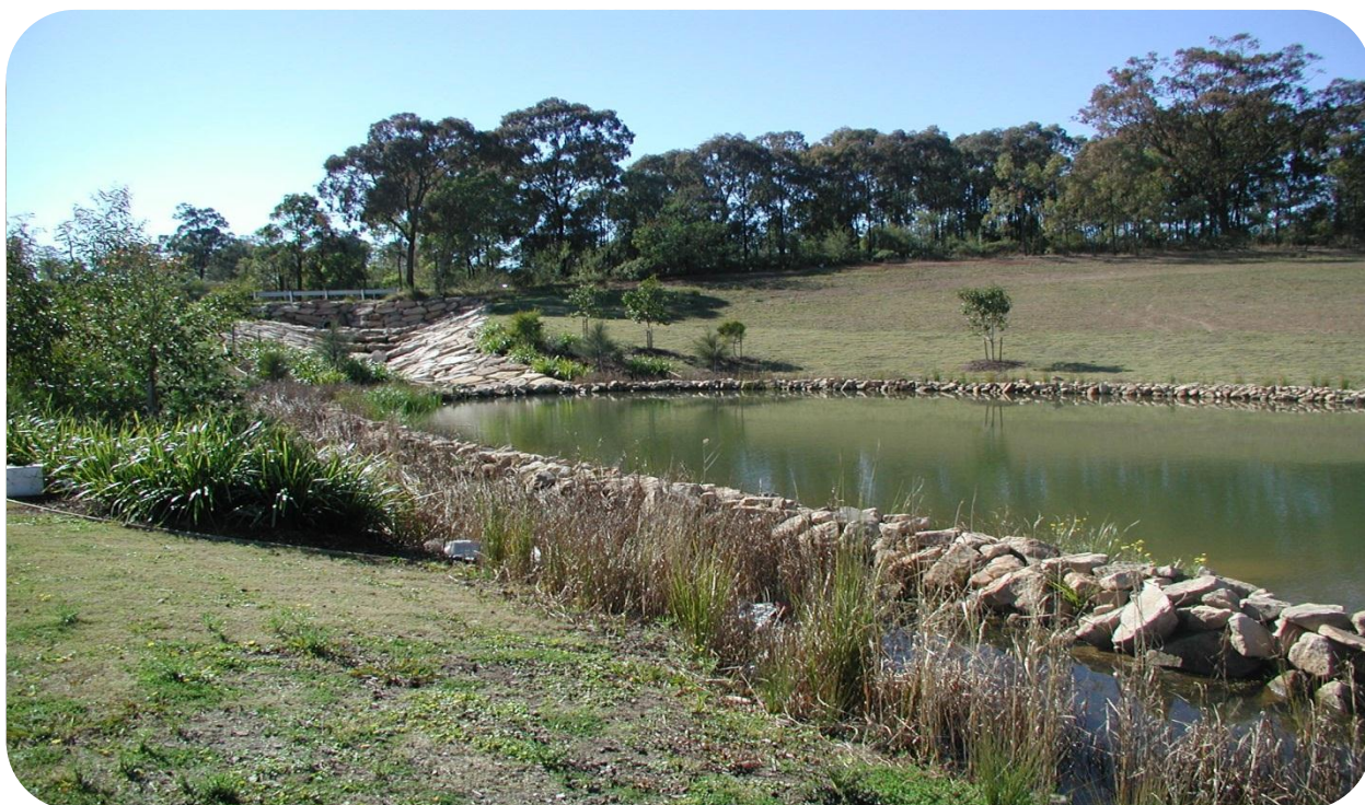
This wet basin collects stormwater to help reduce flood risk to local properties
