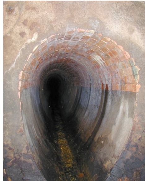
b: Sydney Water Tank Stream Brick Oviform Section
