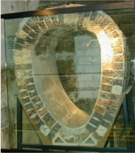
a: Double brick oviform section
