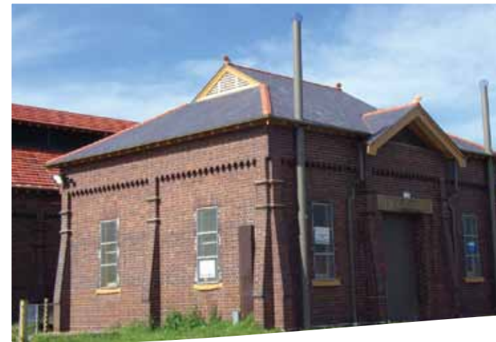
Sewage Pumping Station No. 38.
