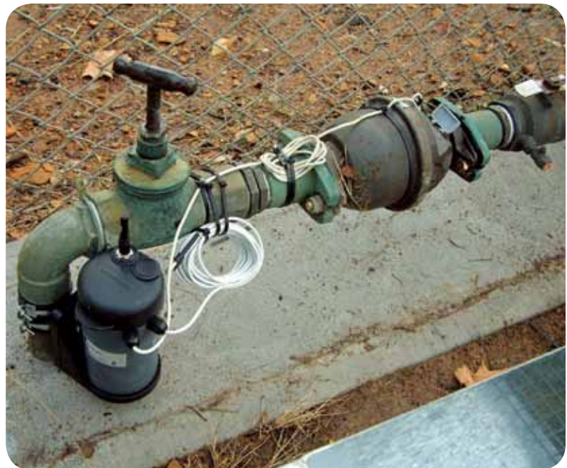
By attaching a data transmitter to a water meter, you can send data to a website
