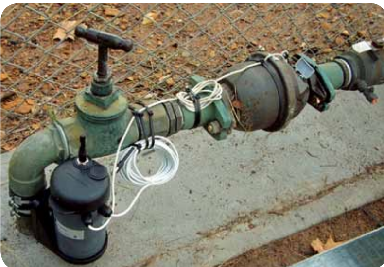
Figure 37 – By attaching a data transmitter to a water meter, you can send data to a website
