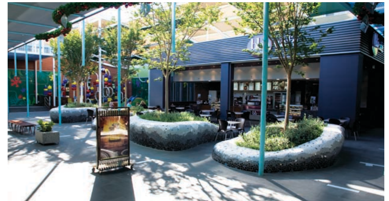
Photograph 8 – The gardens at Rouse Hill Town Centre, owned and managed by The GPT Group, were designed and constructed with water efficiency as a high priority. The site aims to use 60 per cent less water than a typical, equivalent sized shopping centre.
