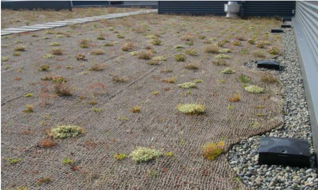
Figure 6-24 EOC Seattle Green Roof (Taylor Associates, 2012)
