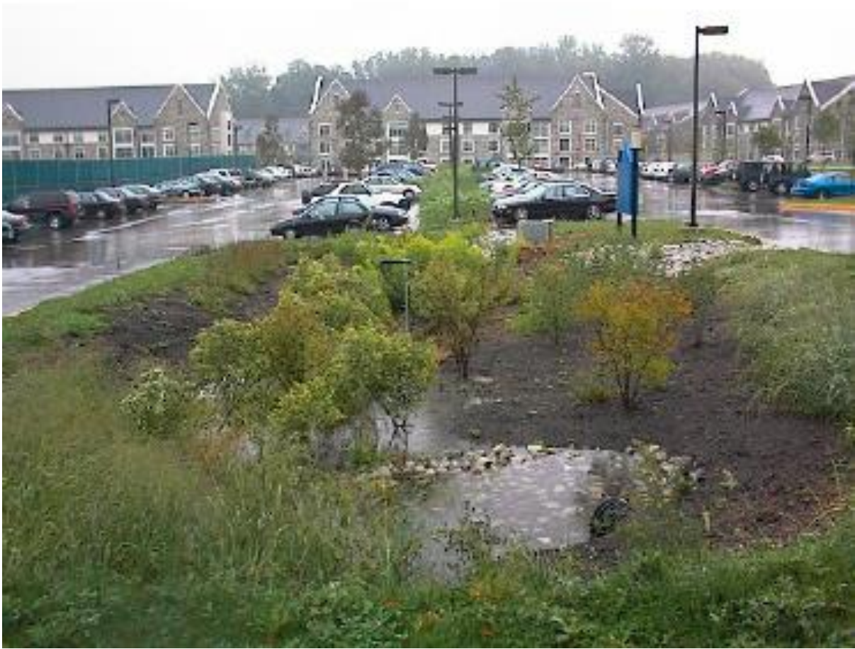
Figure 6-19 Villanova Traffic Island Bioretention (VUSP, 2017)
