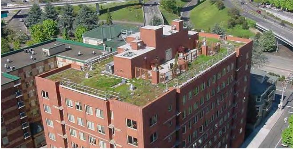
Figure 6-23 Hamilton Ecoroof (Portland Bureau of Environmental Services, 2010)
