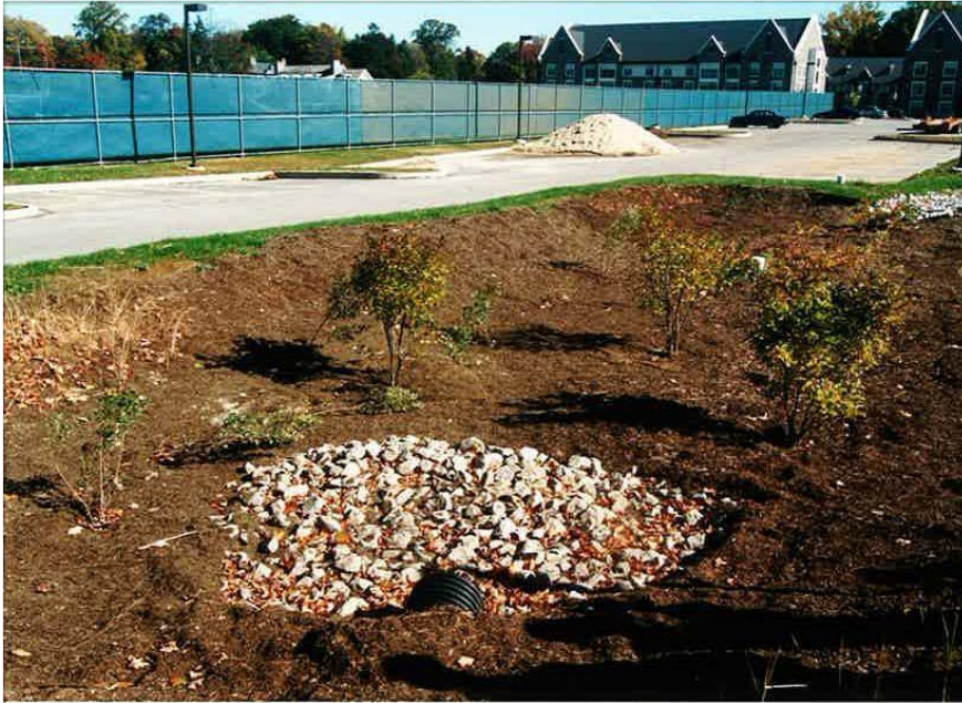
Figure 6-17 Villanova Traffic Island Bioretention (Lord, 2013)
